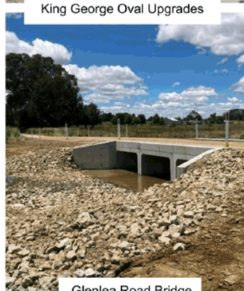
Glenlea Road Bridge
